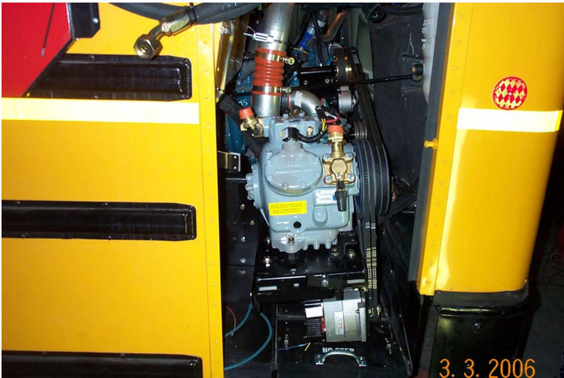
Install Compressor Mounting Plate, Compressor, Tensioner, Alternator and Belts as per drawing. Run Compressor and check pulleys and belts for alignment.
