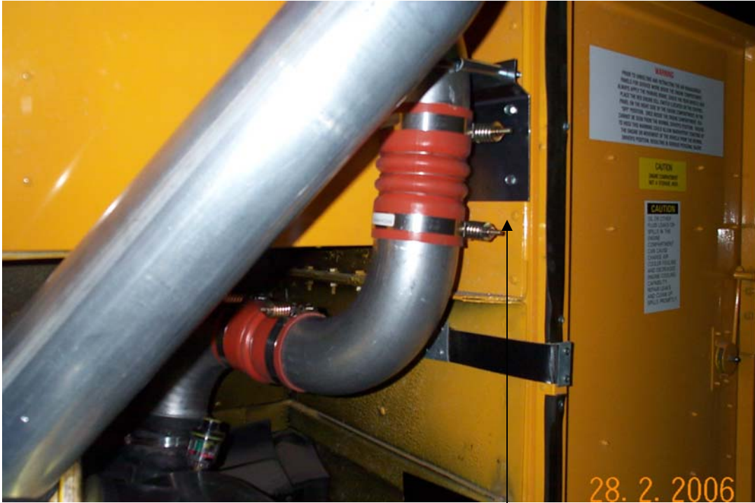
Bracket BMN80026 supplied in kit see Mount Drawing
