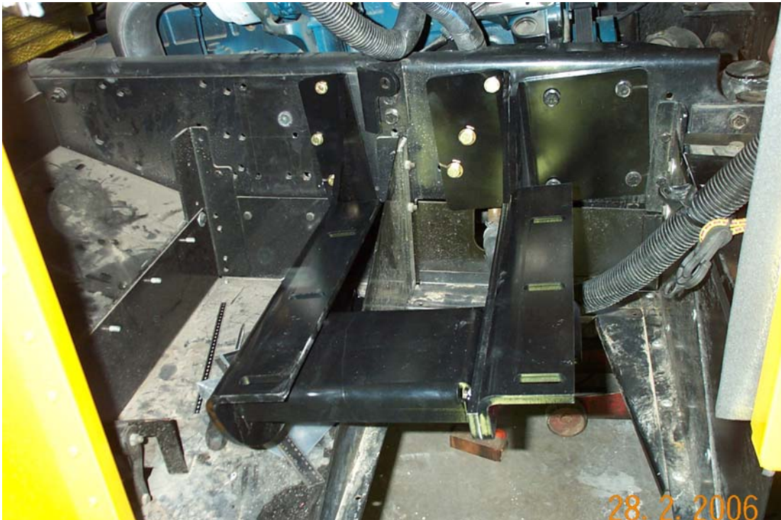
Install Main Compressor Brackets as per drawing.
