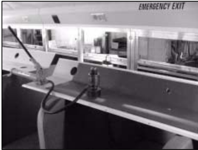
Figure 2-27 Punching out Louver Holes
