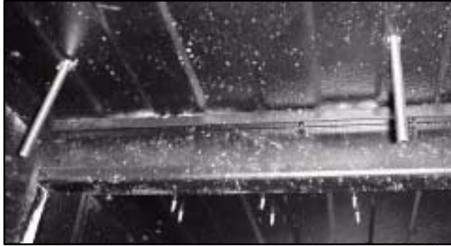
Figure 3-1 3/8 Inch Carriage Bolts Thru Floor
