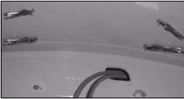
Figure 2-8 Locking Pliers Clamped to Carriage Bolts
