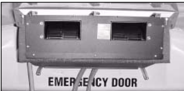
Figure 2-10 Evaporator Mounted to Flat Ceiling
