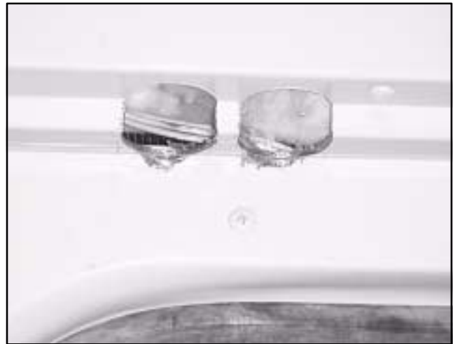
Figure 4-6 Rear Wall Access
