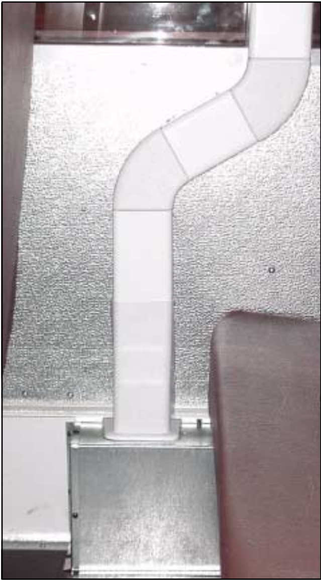
Figure 2-32 Side Mounted Hose Routing (Using 45° Angles)
